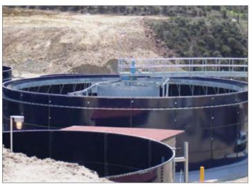
Glass-Fused-to-Steel tanks have a very high resistance to chemical corrosion and have excellent abrasion resistance properties, making them a suitable consideration in your sewage treatment application.
